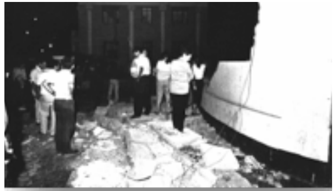
ILD offices destroyed.
